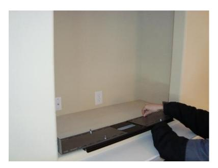
The adapter plates are secured with 8 Carriage bolts (Don't over tighten the carriage bolts, we will have to make a slight adjustment later) that can withstand the force of 400 lbs. Just secure the locking nuts on each bolt and you are ready. Make sure you install the bolts as pictured or the thread from the bolts will get in the way of the TV bracket! (Should be smooth side faced out with the bolts out the back of the mount)
